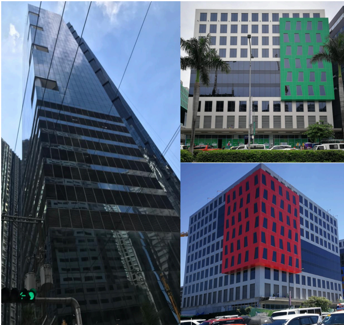
New Office Towers Completed in 2019. Clockwise Left to Right : Jollibee Tower, DoubleDragon Center West, DoubleDragon Center East
