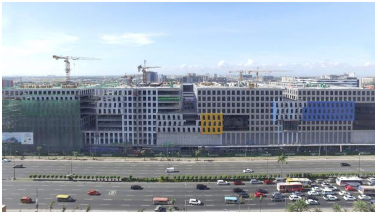
Above: Latest Construction Photo of DoubleDragon Plaza
