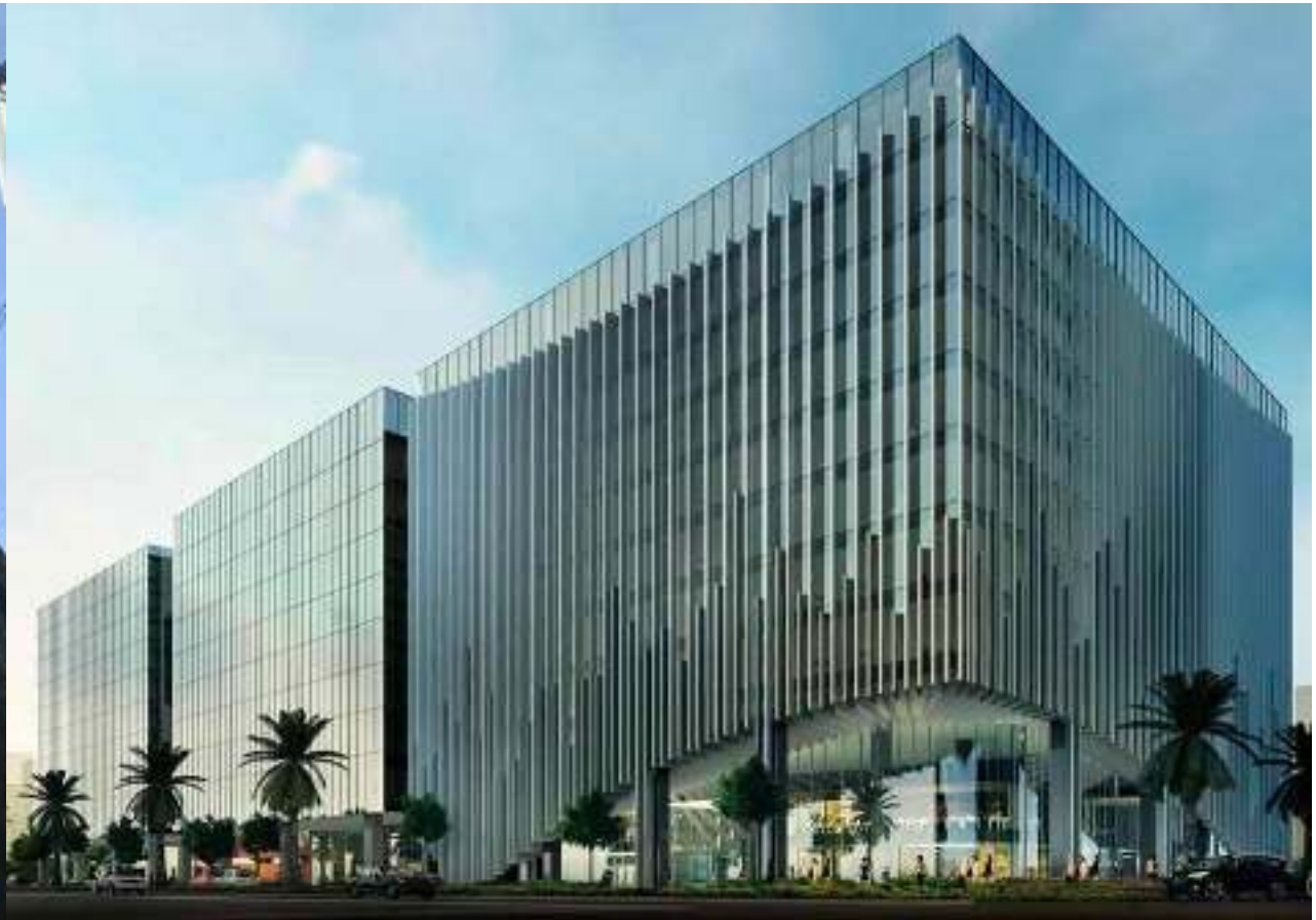
DD MERIDIAN TOWER (DD Meridian Park – Bay Area, Pasay City) Expected Completion 2022
