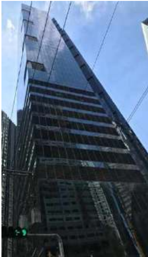
JOLLIBEE TOWER (Ortigas Central Business District)
